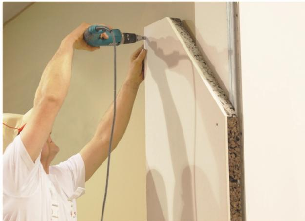
Figure 2: Application of the GYPCORK board.
